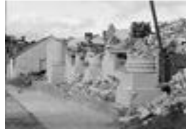
Olympic Theatre demolition-AE2805-67a
